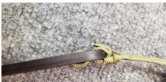
The other end of the antenna wire is secured to another insulator along with the corresponding length of paracord outlined in the plans (diagram above and below). The knot for the paracord was a square knot looped through two holes on the insulator, and the wire was secured as directed by the DX Engineering plan:
